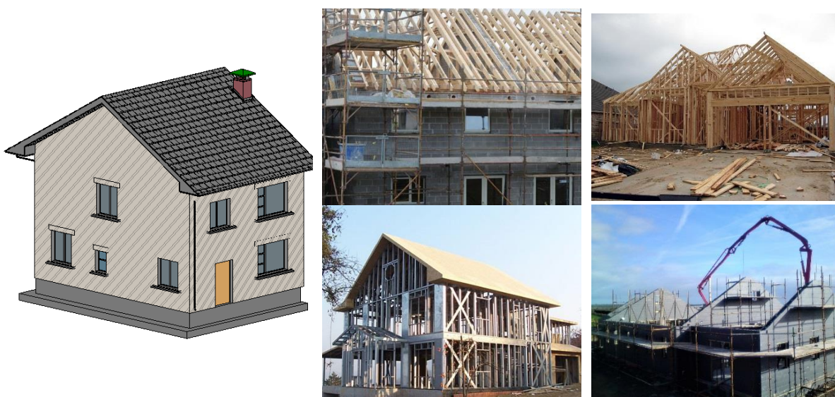
Figure 1: Theoretical semi-detached case study building and the four modern methods for constructing Irish residential buildings to be examined: concrete cavity wall frame, timber frame, light weight steel frame and insulated concrete formwork frame.
